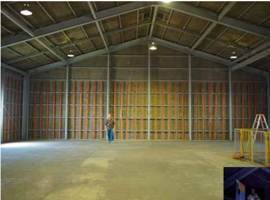
JOEL AND THE FUSHIMI WAREHOUSE
